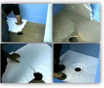
sections are installed into the desired pan area. Walk over the pan sections to help ensure that each piece is fully embedded into the thinset mortar.
