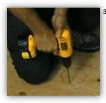
b. Drill Pilot Hole on the inner circle you have hand drawn Use the jigsaw to cut hole in subfloor using the inner-most circle as a guide (~4" diam.). There should be enough clearance for the tail-piece of the drain flange, but the base of the flange is preferably supported by the subfloor. Be sure to (test) dry fit drain flange and pan pieces.
