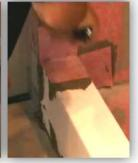
Use your corner-installation techniques to install these at each end of the curb. Finally, measure and cut a proper sized piece of membrane to cover the curb. Ensure that there is a minimum of a 2" overlap onto the pan floor. Install like other membrane sections.
